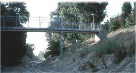
Near **Cheviot Hills**, trains and bicycles would pass under traffic on Overland Avenue for **safety and quiet** (as specified in MTA Phase I EIR, 1994). This extends the existing trench (left) that isolates the right-of-way from neighbors.
